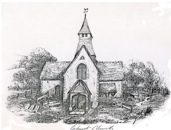
The church of St Peter & St Paul, Ewhurst before the collapse of the tower in 1837
